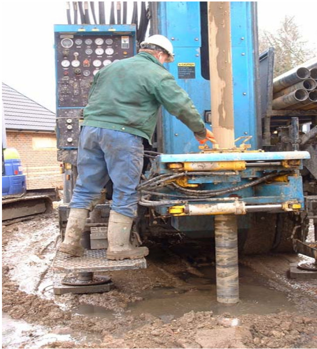
Installing ground source heat pump
