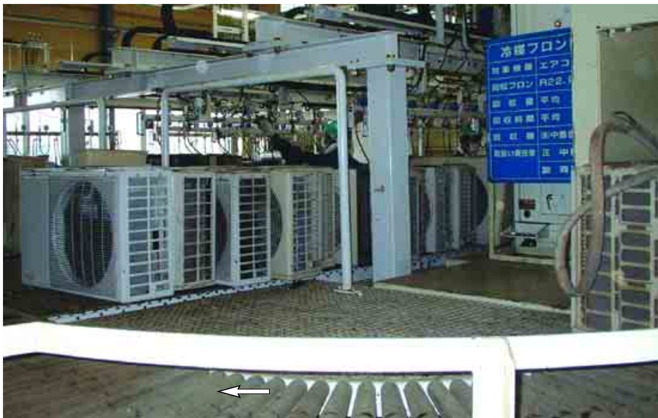
Exhibit D.26 Conveyor system with air conditioners ready for processing at Green Cycle plant (arrow indicates rollers necessitating manual intervention to enable movement of units)
