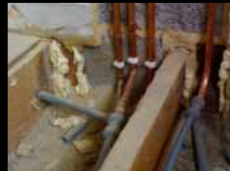
Sealing up all holes Air tight home
