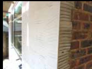
30 mm insulating exterior render
