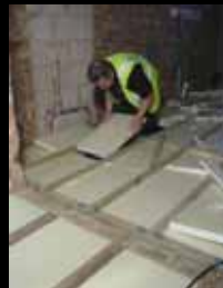
40 mm under floor insulation
