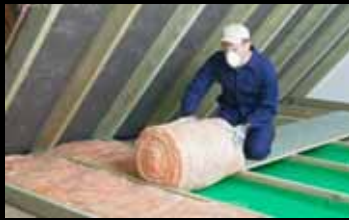
270 mm grant assisted loft insulation
