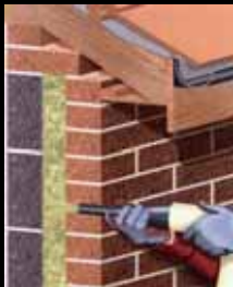
Cavity wall insulation Grant assisted
